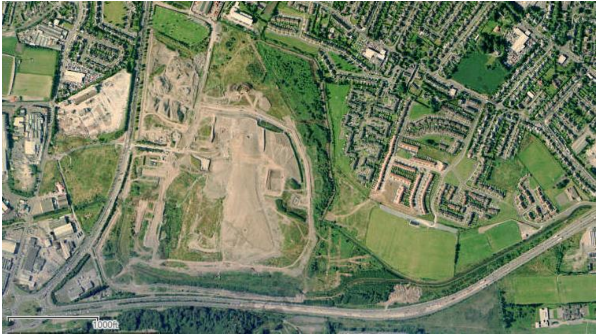
Figure 2.20. Aerial photograph of Tramore Valley Park when it was in use as the Kinsale Road Dump (1999).
