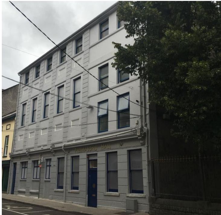
Figure 4.4. Photograph of Freemason’s Hall on the left and a section of Bishop Lucey Park on the right.
