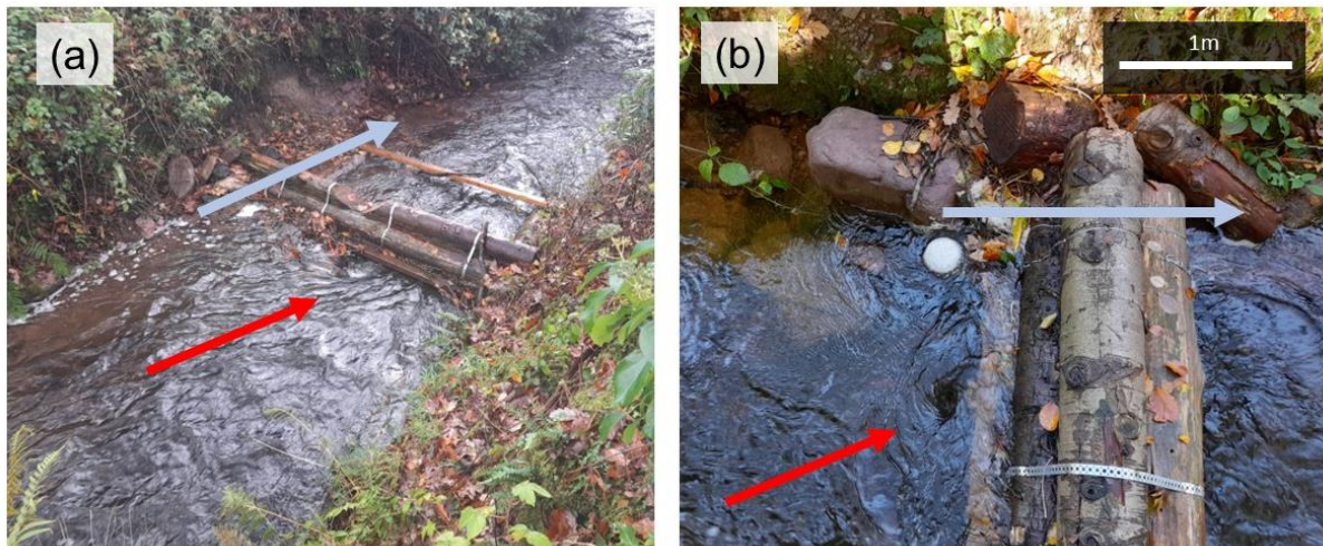
Figure 7 Photographs of leaky dams with red arrows indicating locations of streambed scour induced beneath leaky dams. Blue arrows indicate direction of stream flow. Partial blockage by woody debris of the most upstream leaky dam (Fig. 7a) causes downwelling and high flow velocities through the freeboard beneath the leaky dam. High flow conditions in Fig. 7b cause eddying of water on the upstream side of the leaky dam and consequent localised erosive forces on the streambed. 1m scale is shown at top right of Fig. 7b.
